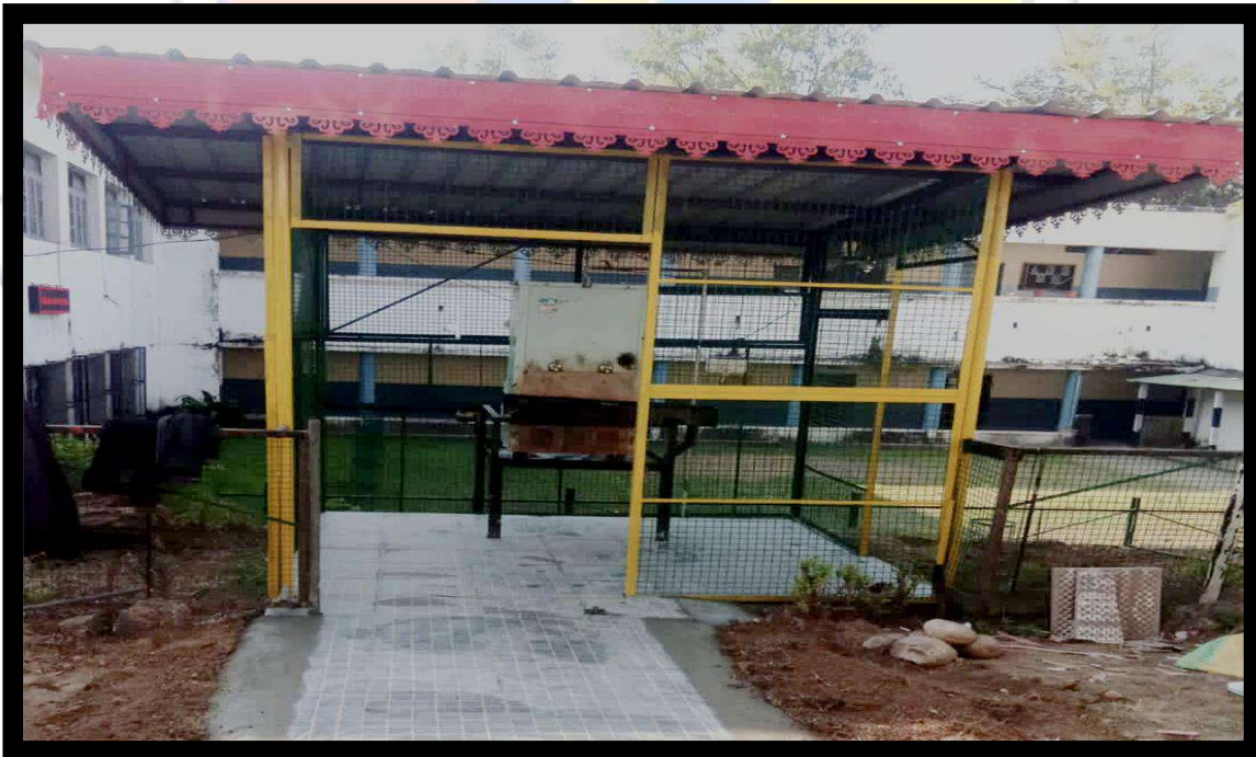
SHADED WATER COOLER FACILITY
